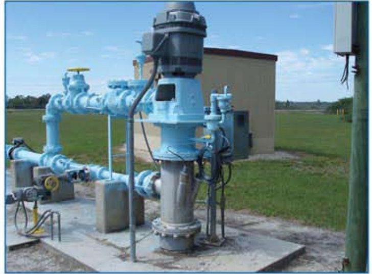
Monitoring recharge rate in an aquifer storage and recovery (ASR) project using Level TROLL 700
