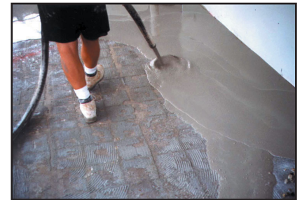
Self-leveling underlacements.
