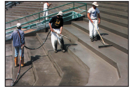
Concrete resurfacing.
